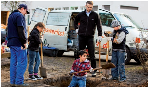
Erecting a climbing frame for a remedial school as part of a TeamACTIVE project
